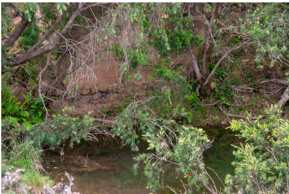
Figure 8: Pier base in small creek at underbridge. The founding of this pier needs to be checked against drawings and rip-rap may be needed to limit future risk from scour.
