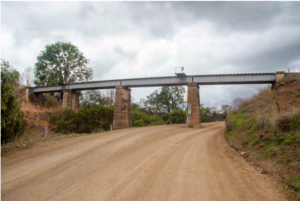
Figure 6: Underbridge north of Kalpowar. The bridge uses welded plate web girders, which may be a modern replacement for an older superstructure as such girders were not used at the time of the original construction
