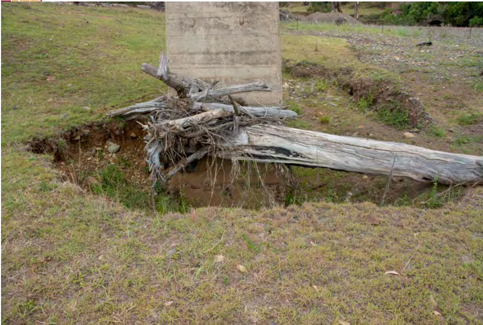
Figure 9: Scour around pier base at Glassford Creek. If the pier is founded soundly on rock, risk is low. Otherwise rip-rap could be dumped to limit further scour.
