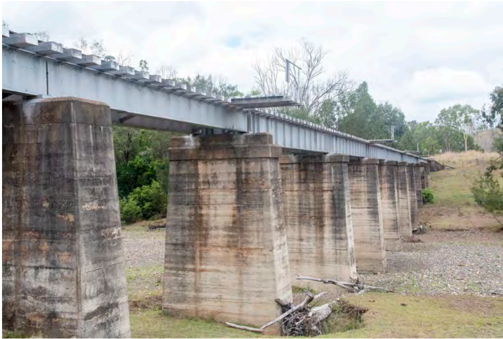
Figure 7: Glassford Creek bridge. The superstructure of the centre seven spans are made from rivetted plate web girders; three spans on each end use compound girders with flange plates rivetted top and bottom. Changes in the pier tops also suggest that the bridge was lengthened after the original construction.
