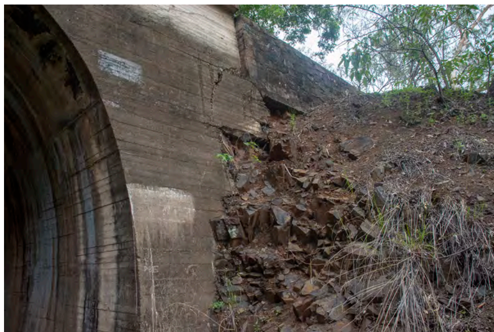
Figure 4. The northern portal of Tunnel 4 has had the wingwall extended using a wall built from stone. This wall, which may have been an informal solution by the builders has moved from earth pressure and broken the concrete to which it was attached.
