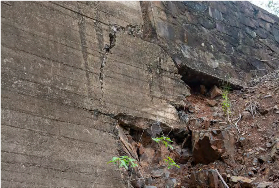
Figure 5. Detail of figure 4. It can be seen that the stone wall on the right has possibly moved outwards and its base undermined. The movement has taken part of the concrete headwall with it.
